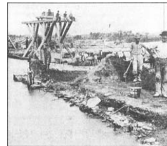
Photo of excavation for Mill #3 construction
