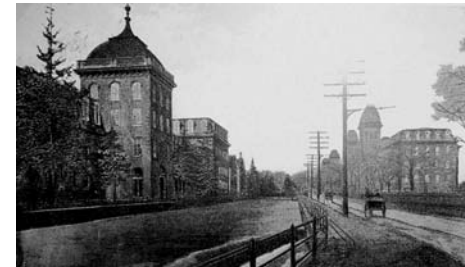
Postcard view of North Mohawk Street. Harmony Mill #3 is on the right, and Harmony Mill #2 is on the left. The waterway in front of Mill #2 is the original Clinton's Ditch, converted to a power canal for the mills.
