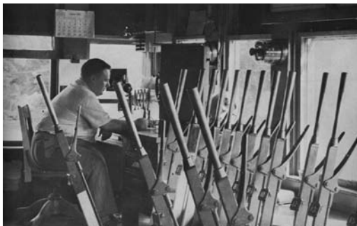
Towermen controlled the shunting of rail cars mechanically from the control tower. (Mechanicville City Historian)
