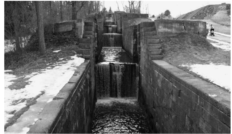
"The Flight" (today called "The Combine") is a series of five locks on the Glens Falls Feeder Canal in Fort Edward, which raised/lowered canal boats a total of 55 vertical feet. (Wikipedia)
