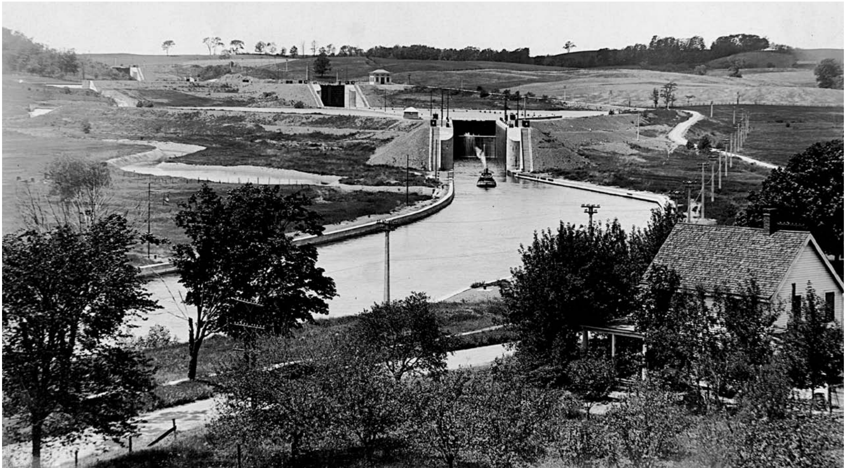
Built in 1907, the Waterford flight of locks raises watercraft 165 feet, from the Hudson River to the Erie Canal, in just over a mile. (New York State Archives)
